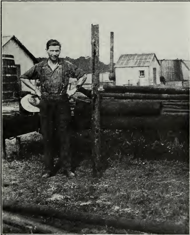
Fig. 20. Photograph of a casing corroded by water in the Flat Rock Pool.
